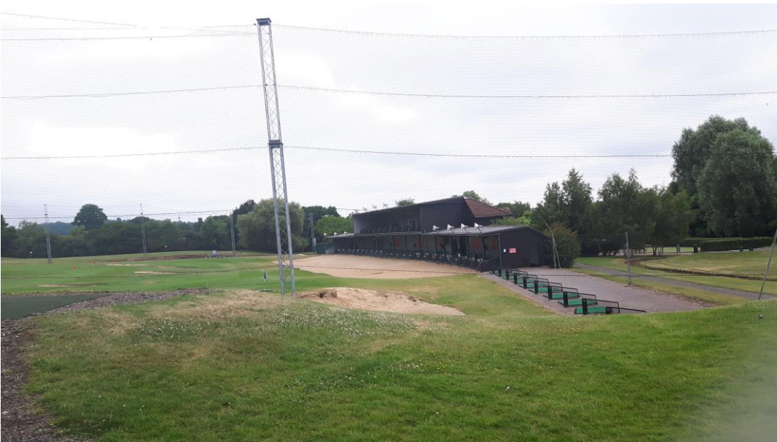
Rear elevation and driving range bays with metal pylons
